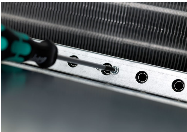
Figur 10. Injustering, dysa, M
