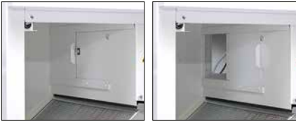
Bypass past the heat exchanger: The cover closed in the winter; open in the summer.
