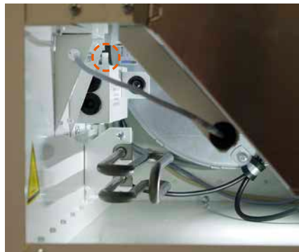
Reset button for the overheating protection on the preheating air heater(Only models with electric air heater)
