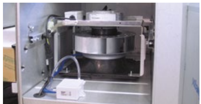
Direct-driven fans with EC motors.
