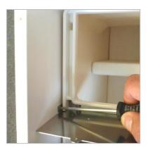
6 Seal the gap between the wall box and the telescoping adapter air and water prove.
