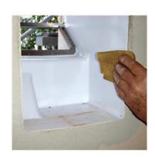
5. Support the appliance with your right hand in front and bottom and slide it straight into the box. Slide by pressing the front panel on the unit until it stops.
