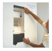
3. After inserting the device, the cover is inserted into the four detent plates and pressed against the wall.
