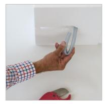
2. Seal the remaining opening in the BOX with sealing tape airtight.
