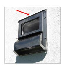
13. Hook-in the outside hood and attach with 2 M4 raised head screws.
