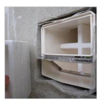
4. Shorten the telescopic adapter in case your wall thickness (including plaster) is less than 45 cm.
