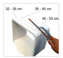
5. Install telescoping adapter flush with stucco. Use water prove sealant as shown.
