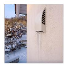
1. If you cannot connect the condensate drain, first cut the hose and then stow it safely.
