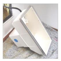
7. After the wall cut-out is completed install the electrical cable (3 x 1.5 mm²) in the upper part of the wall box. Affix the wall box flush with plaster, perpendicularly and secure with wedges.
