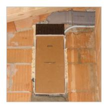
10. Push in the finger tabs to remove box bracing.
