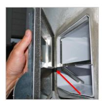
12. The metal outside air divider is attached to the telescoping adapter via 6 metal screws.
