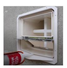
7. In addition, seal the gap between the wall box and the telescoping adaptor water prove to the required level with the enclosed sealing tape.
