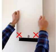
2. Push the two metal flaps apart and remove the dirty supply filter.
