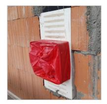
2. Remove the protective cover from the outside cap after all plaster and painting work is done.
