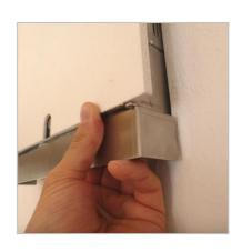
2. Attach the metal sheet using two M3x5 raised head screws.
