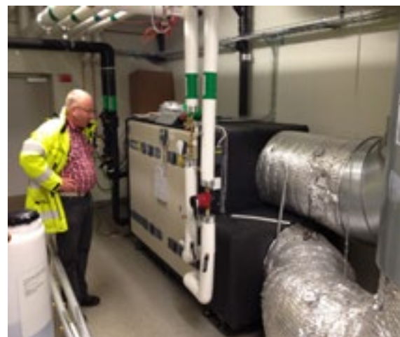
Technician Björn Adler inspecting a GOLD air handling unit. Photo: Swegon
