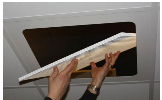
Figure 2. RASTER installation in ADAPTER.
