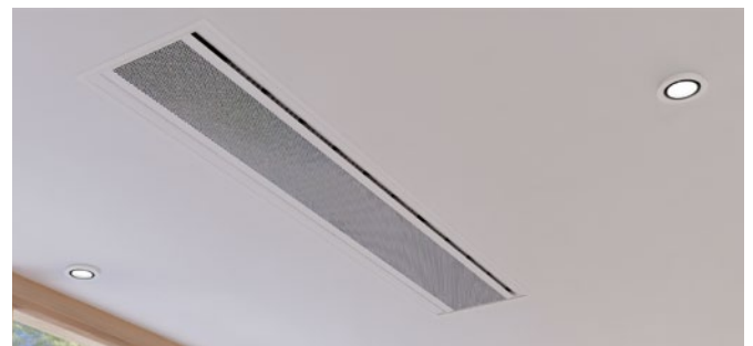
Figure 9. REACT Pacific with Plasterboard frame, PACIFIC T-FPB
