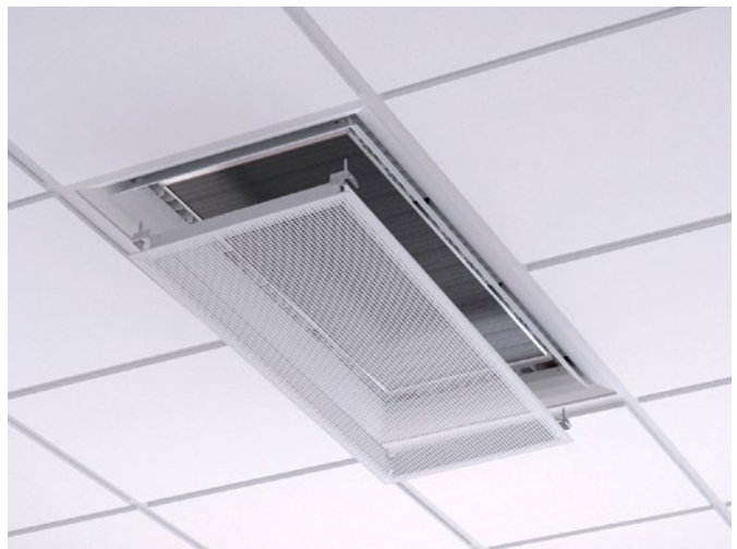
Figure 10. Removing the face plate to access the coil
