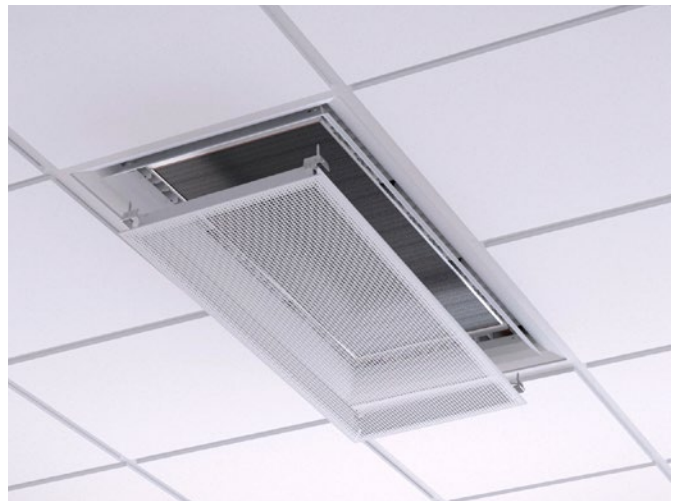
Figure 17. Removing the face plate to access the coil
