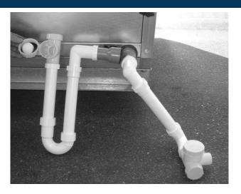
The siphon height should be accurately determined, dependent upon the pressure head.
