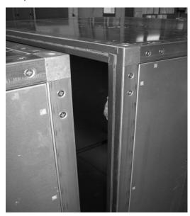
Winch the equipment components together until they are positioned exactly together
