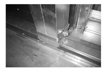
The section points of the outer equipment components are to be subsequently sealed with the sealing compound as provided.
