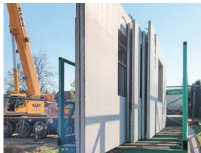
No restrictions when loading the trucks, because the bare brickwork set is inserted flush
