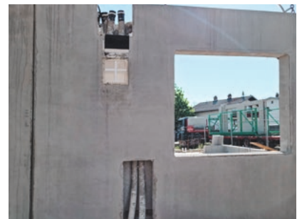
Placement of the prefabricated wall including all ducts
