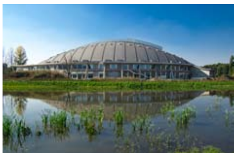
Pruszków Velodrom, Poland Arena Solution
